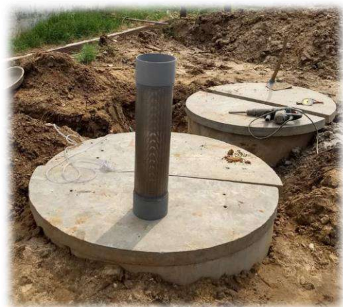
Installation of V-wire technology
