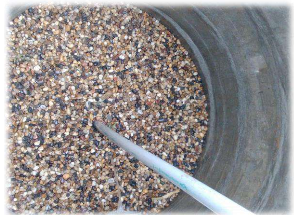
Gravels and clay packing filter
