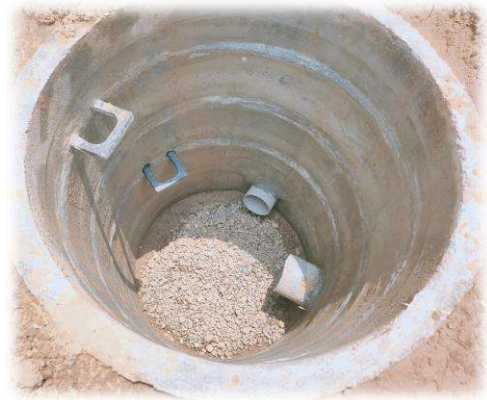
Silt trap connected to storm water drain
