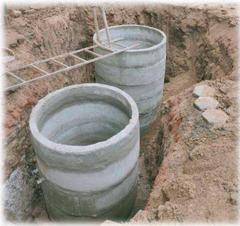
Recharge well and silt trap
