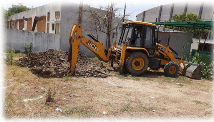
JCB digging the water collection pit
