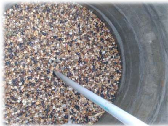
Gravels and clay packing for filter.
