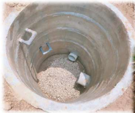
Silt trap connected with drain and Storm water drain.
