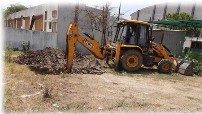
Pit digging with JCB for water collection for construction.
